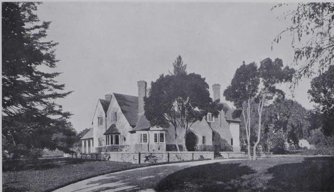
THE DOVER, POLING, NEAR ARUNDEL, SUSSEX. THE LOWER PARTS OF THE WALLS ARE FACED WITH RED BRICKS OF VARIED COLOUR, WHILE THE UPPER PART IS COVERED WITH CEMENT ROUGHCAST
