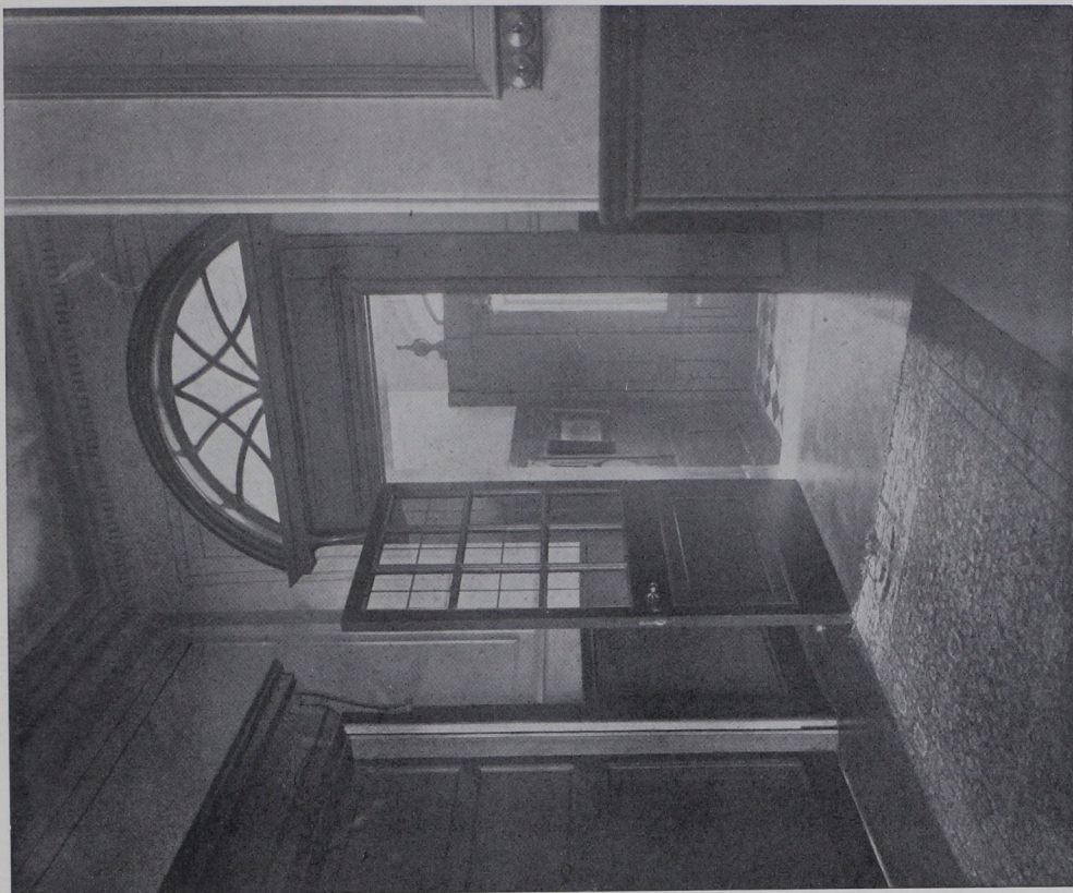
VESTIBULE AND ENTRANCE HALL, KINGSBURGH GARDENS, GLASGOW.
