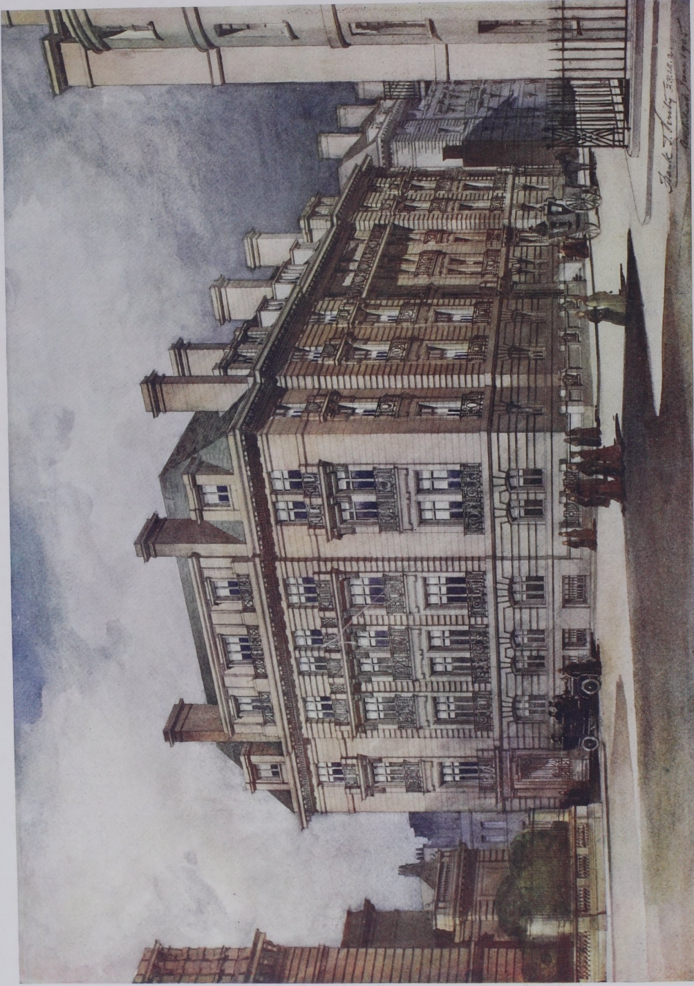
FLATS AND MANSIONS, CLEVELAND ROW, ST. JAMES'S, LONDON, S.W. MATERIALS: PORTLAND STONE, FRONTS "GREEN SEDAN COUNTESSE," THE ROOFING OF SLATES. THE HEIGHTS OF THE HORIZONTAL LINES ARE GOVERNED BY THE MAIN HORIZONTALS OF THE NEIGHBOURING PROPERTY; THE WINDOWS, GROUPED SYMMETRICALLY, ARE ENRICHED WITH IRON BALCONIES
