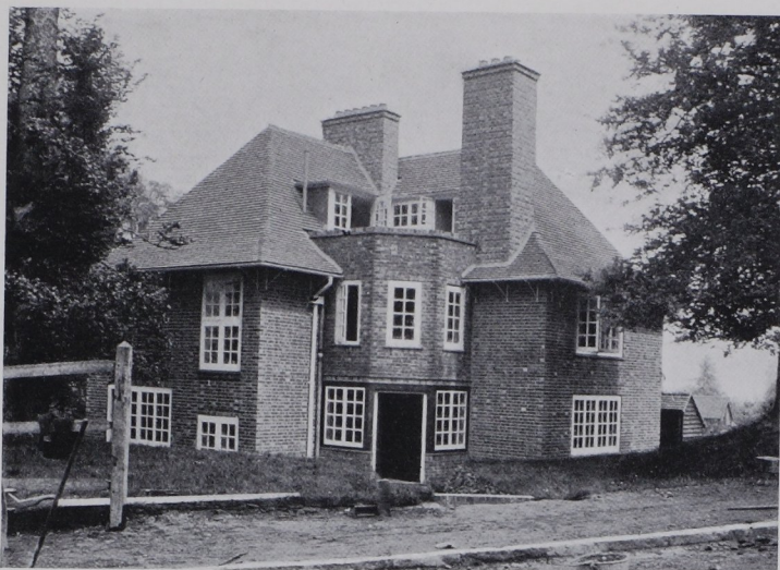
SPRING BANK, WESTCOTT, NEAR DORKING. THE GROUND PLAN OF THIS UNFINISHED COTTAGE IS GIVEN BELOW.
