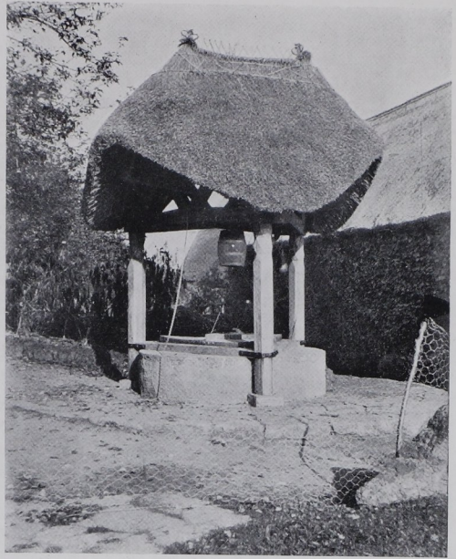
NETHERTON, SOUTH DEVON. THE RAINWATER WELL
