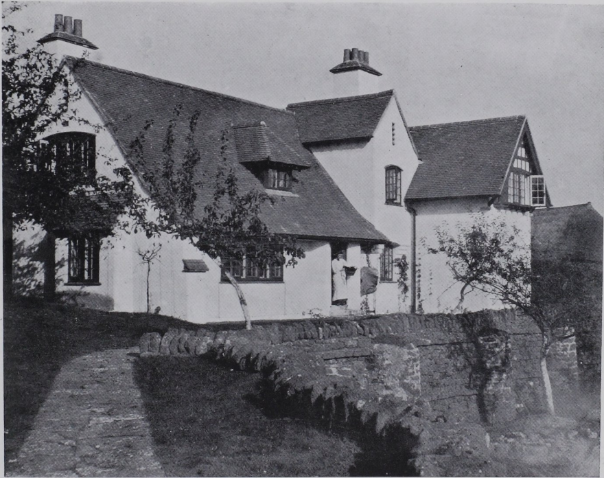
NETHERTON, SOUTH DEVON. FRONT VIEW OF THE COTTAGE SHOWING PART OF THE TERRACE WALL
