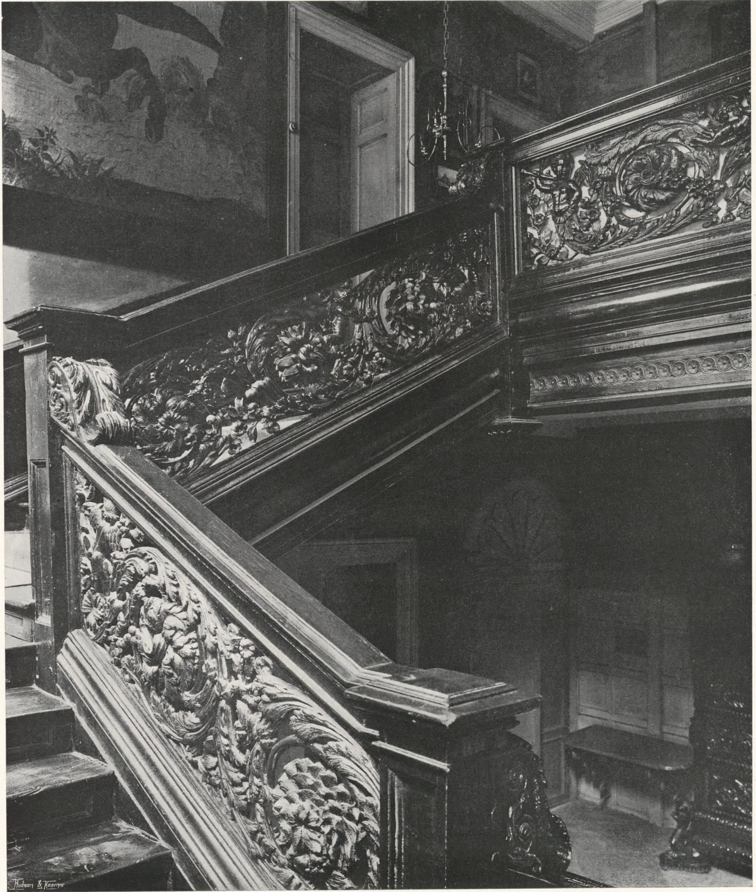
THE GRAND STAIRWAY.
