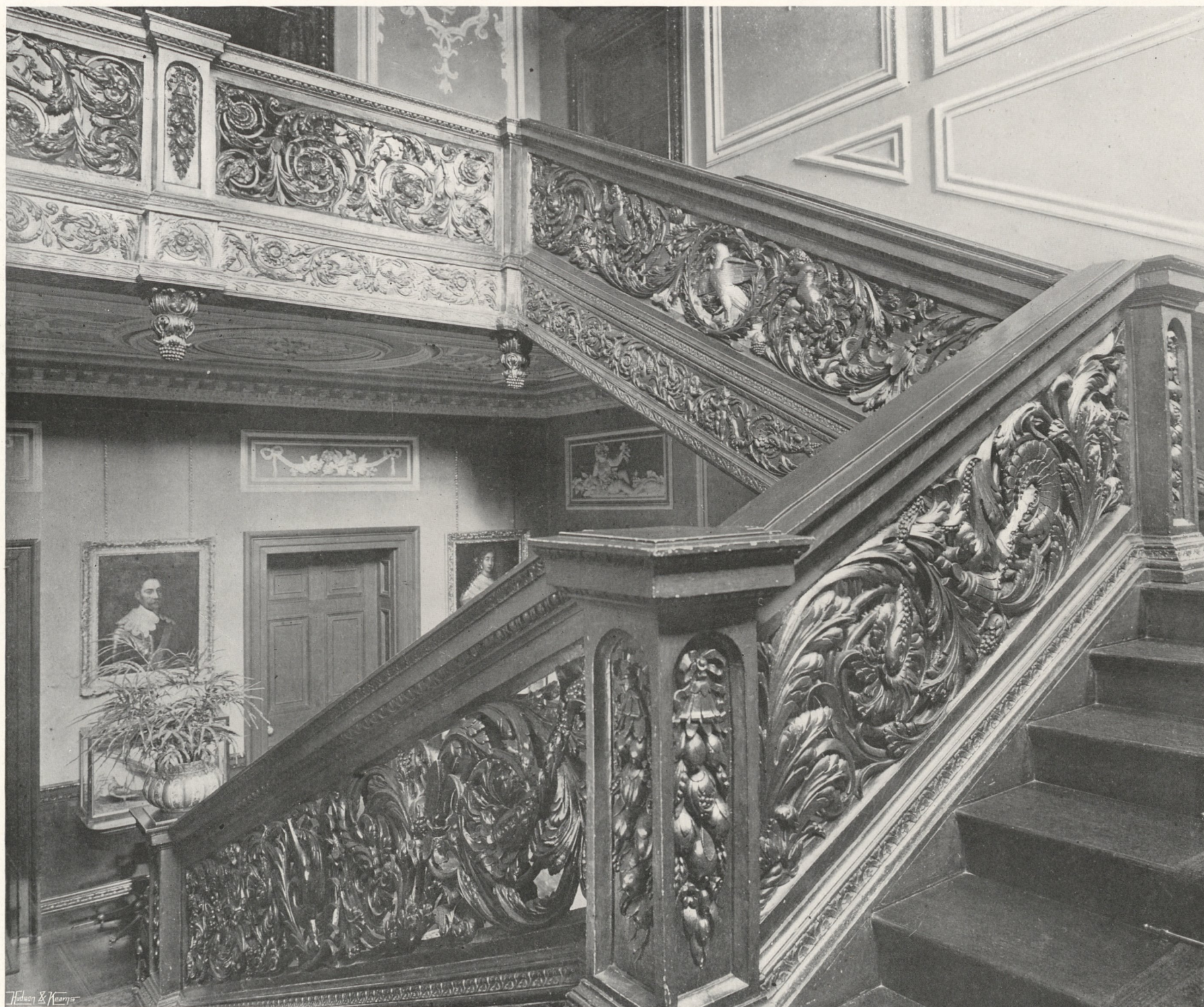
FOUR SIDES OF THE STAIRWAY.
