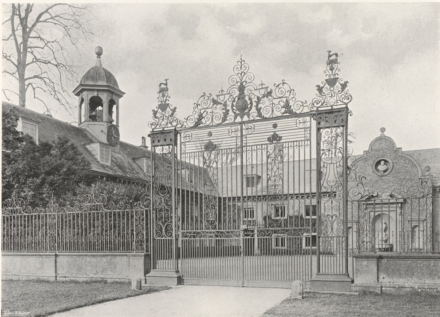
THE WEST FORECOURT,
