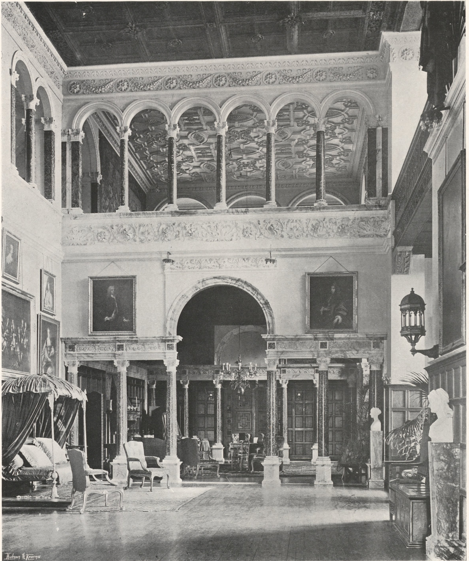
THE SOUTH END OF THE GREAT HALL.
