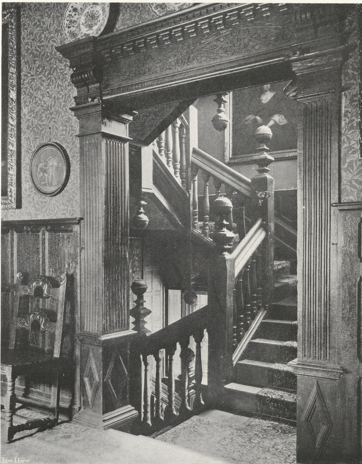
THE SOUTH STAIRCASE.
