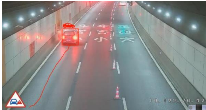
Figure 1: Stopped vehicle in a tunnel, Source: Citilog CT-IM-AID_Functions_specifications-RevL.pdf
