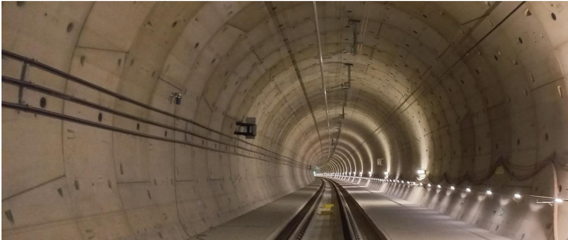
Figure 3: Finish of the tunnel surface
