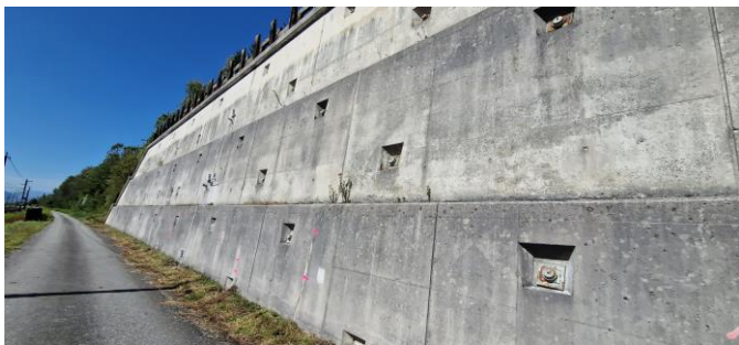
Figure 2: View of the anchor wall.
