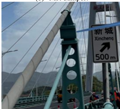
(c) Viscous shear damper.
