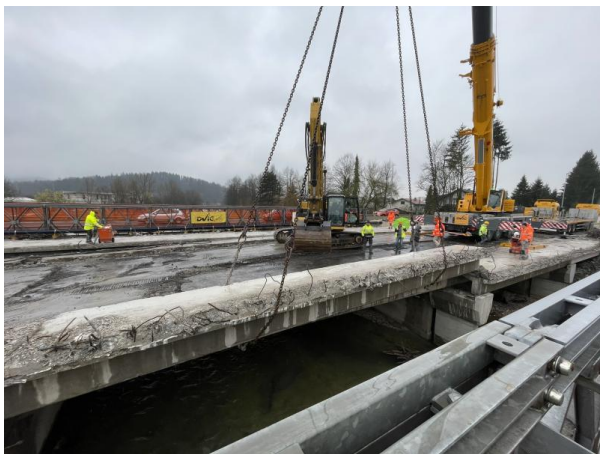
Figure 3. Lifting the girders with cranes.
