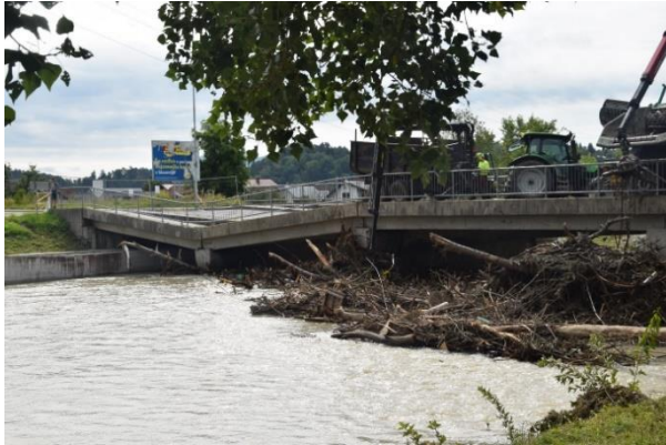
Figure 2. Partly collapsed bridge after floods (upstream).
