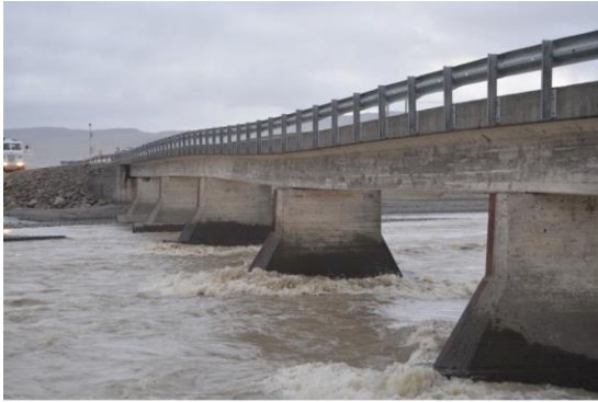
Figure 5. The intermediate pillar of the bridge has sunk [10].
