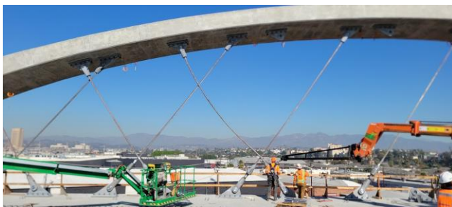
Figure 6. View of typical strand hanging operation
