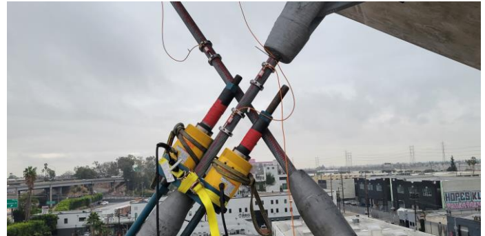
Figure 7. Contractors strand loading system
