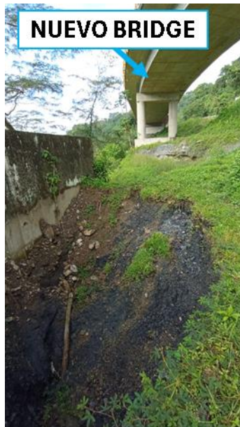
Figure 5. Evidence of mass wasting processes near the foundations of the PR81 corridor bridges
