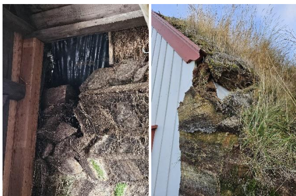
Figure 4: Examples of plastic membranes in turf roofs. Left: membrane visible from the inside. Right: membrane visible from the outside.
