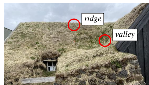
Figure 11: Sensor locations on south side of roof in Keldur.
