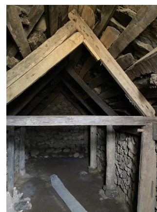
Figure 6: Structural system in the kitchen in Keldur.
