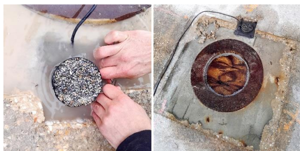
Figure 13. Installation of a moisture sensor on the reinforcement (Copyright: Eugen Kronhardt, Infrasolute).
