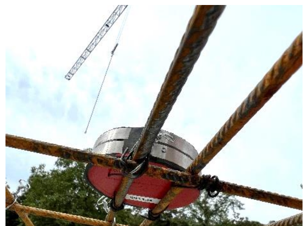
Figure 2. Attachment of moisture sensors in a new construction project using binding wires directly on the reinforcement (Copyright: Christian Steffes, Infrasolute).
