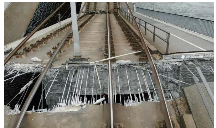
Figure 5. Failed cross-section in axis D with pulled-out steel reinforcement.
