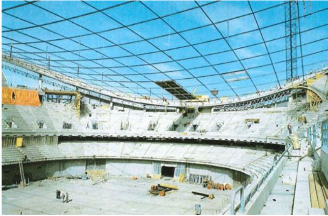
Figure 2. Sagging and Hogging Cables 2
