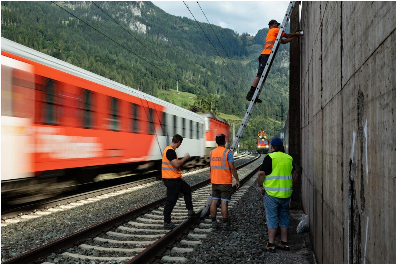
Figure 1 : Installation of tilt sensors for monitoring a retaining wall in a track area with restricted access
