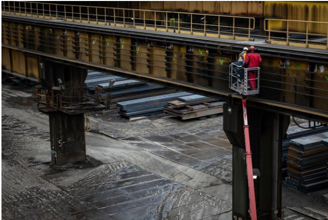
Figure 6: Installation of tilt sensors on the supports and longitudinal beams of the crane rails
