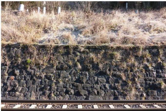
Figure 1. Gravity wall along the Semmering railway line.
