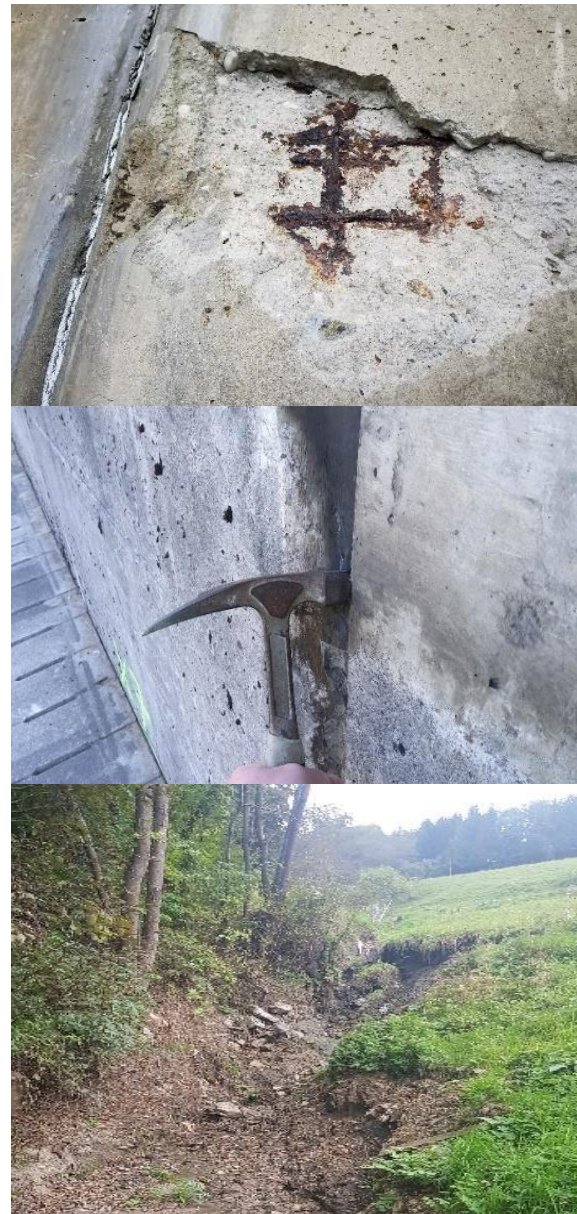
Figure 3. Examples for damages found during inspection of civil engineering structures; reinforcement corrosion and concrete spalling (top); shift and misalignment within a construction joint (center); erosion and unguided surface flow (bottom).
