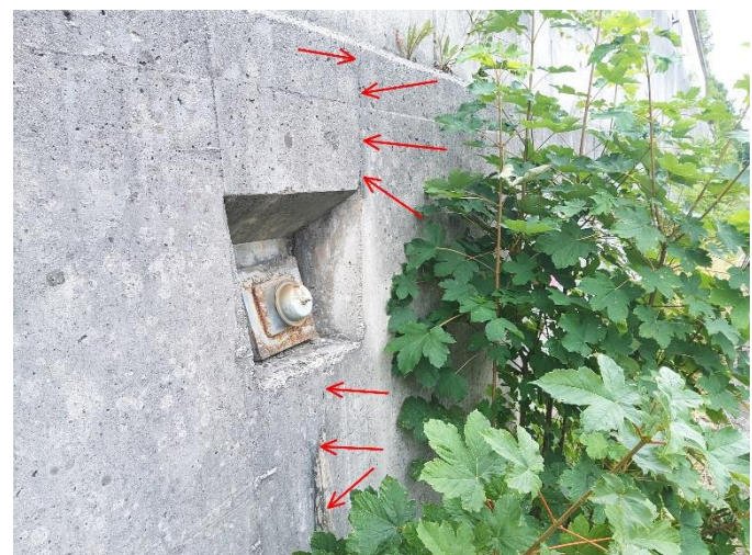
Figure 11. Cracks along the concrete structure and adjacent to the anchors.
