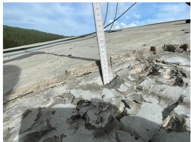
Fig. 3: Damaged area with heavily segregated concrete structure.
