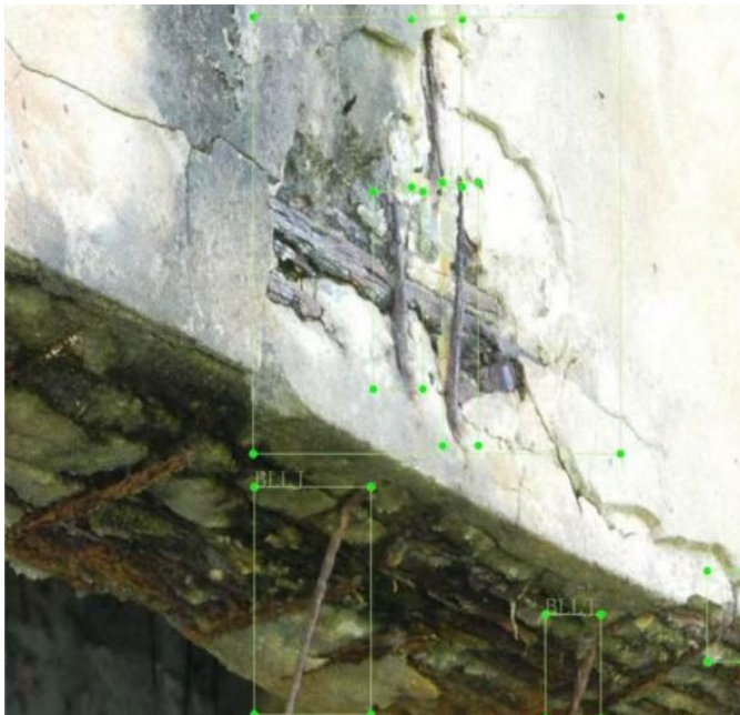
Figure 5. Spalling & Exposed reinforcement.
