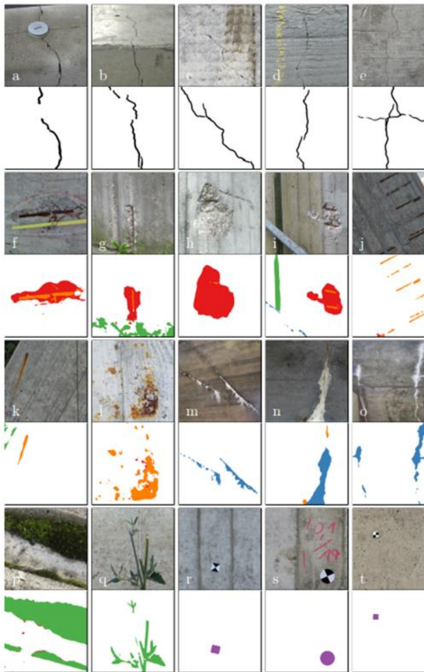
Figure 2. S2DS Classes and Labels: crack (black), spalling (red), corrosion (orange), efflorescence (blue), vegetation (green), and control point (purple) [20]
