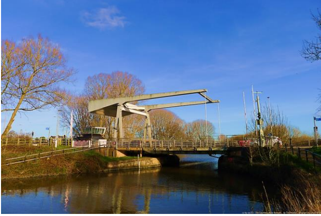
Figure 2. Bascule bridge, constructed in 1972, carrying the A379 over the Exeter Canal in Devon, England, UK.
