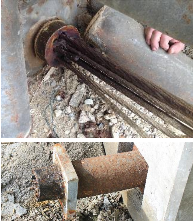
Figure 4. Corroded tension elements of the external parts of strand anchors.
