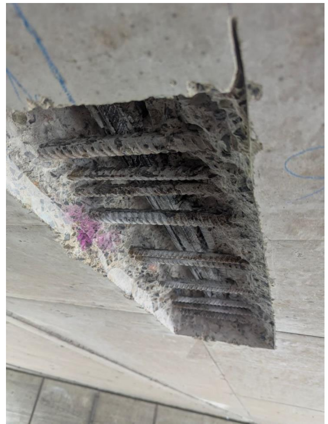
Figure 10. Sampling of prestressing wires from an existing road bridge for material testing (source: LS Brandenburg).
