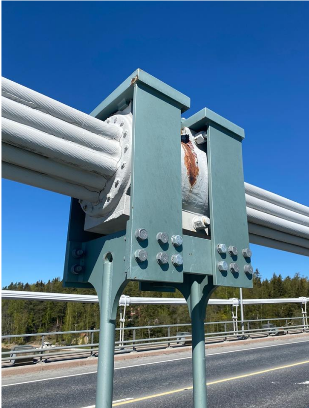
Figure 9. Hanger arrangement resulting in bending stresses due the superstructure longitudinal movement,
