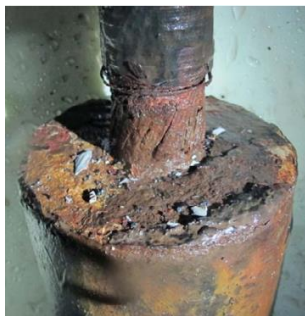
Figure 2. Corroded hanger
