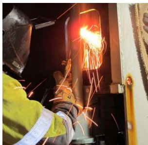
Figure 3. Installation of temporary hanger bars.
