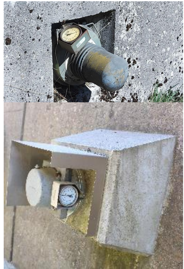
Figure 7. Anchor load plate installed during the construction of the structure.
