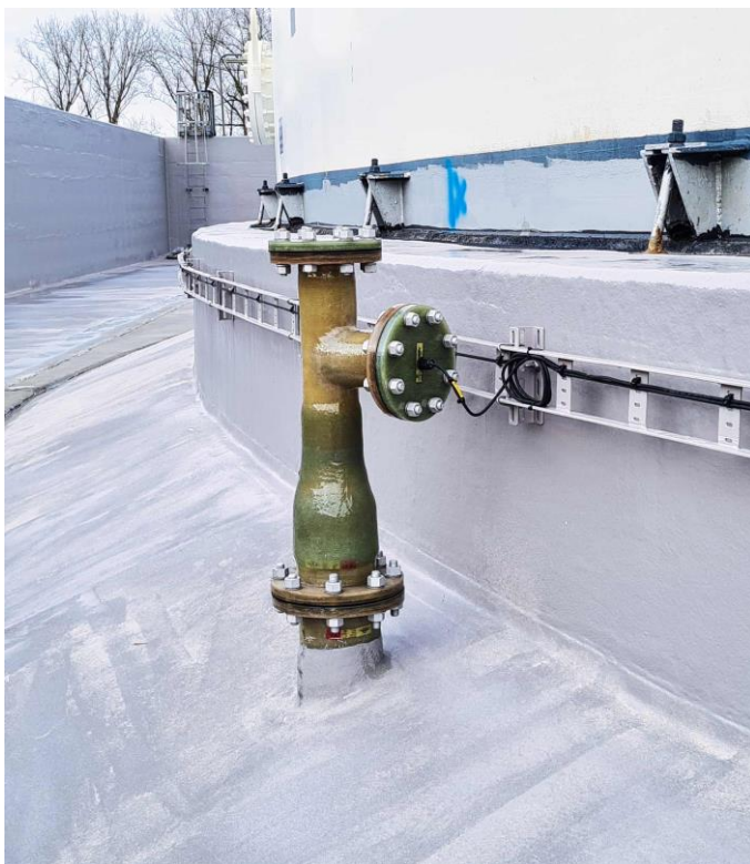
Figure 12. Leak monitoring system with eight sensors embedded around the perimeter of the monitored tank using mounting sleeves.
