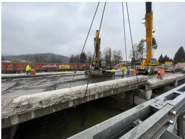
Figure 3. Lifting the girders with cranes.
