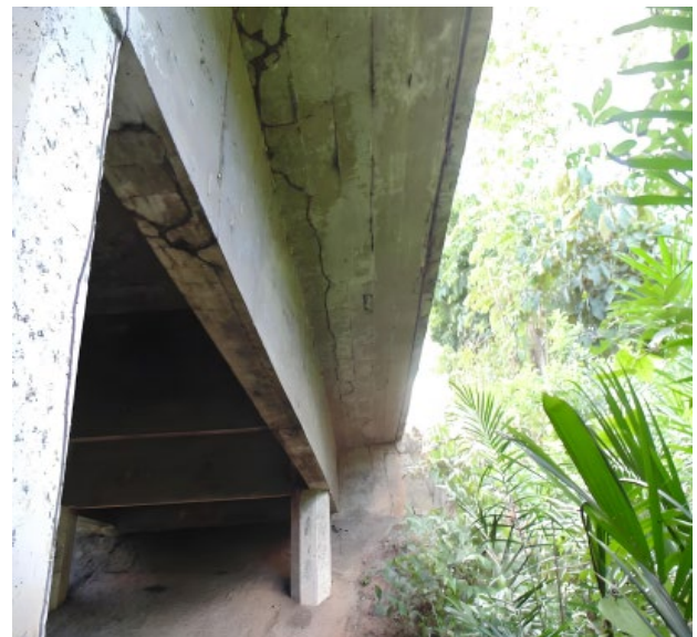
Figure 4. Defects on the bridge.
