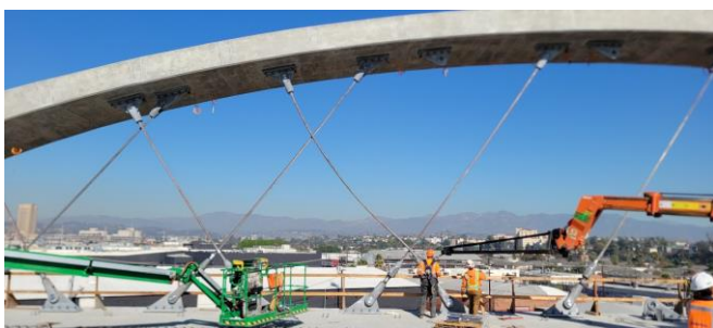
Figure 6. View of typical strand hanging operation
