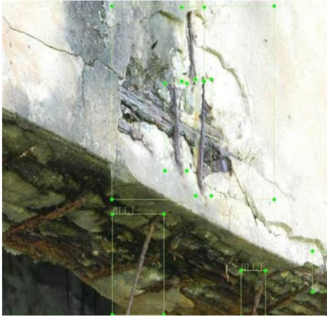
Figure 5. Spalling & Exposed reinforcement.
