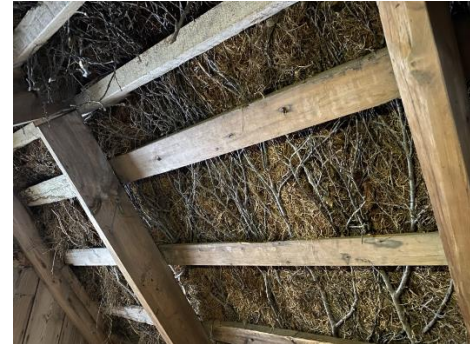
Figure 2: Example of dried birch twigs carried by purlins and rafters (thatched roof).
