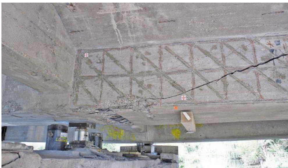
Figure 1 Applied DFOS on the Hammelburg bridge girder web, taken from [6]
