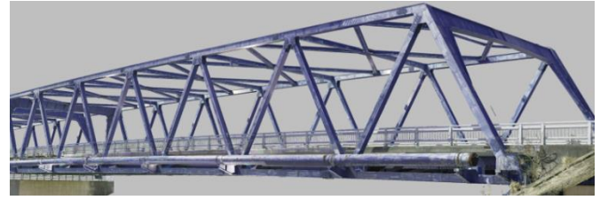
Figure 10. The point cloud data measured with a stationary laser scanner
