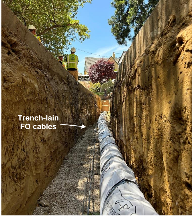
Figure 5. Trench-lain fiber optic cable installation
