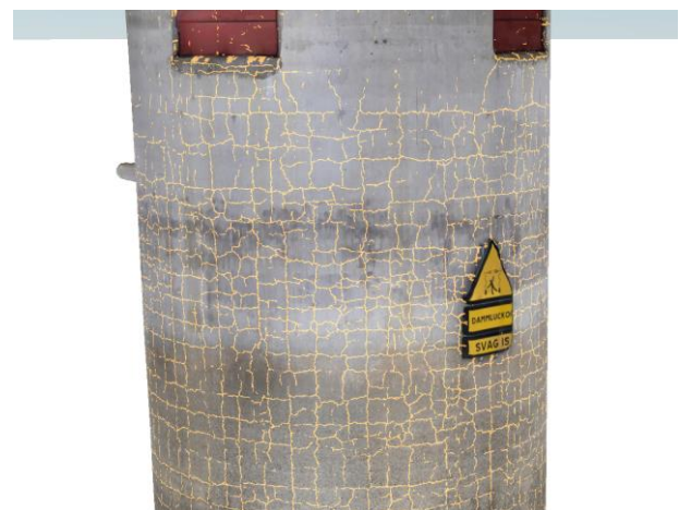
Figure 2. Resulting 3D projected AI interpretation of crack pattern
