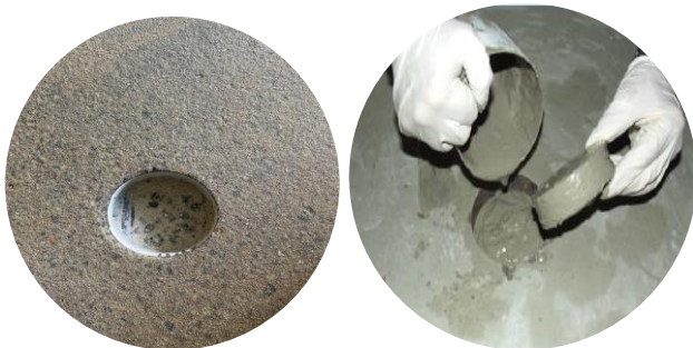
Figure 3. Core drilling with a diameter of 100 mm and installation of the sensor using coupling mortar (Copyright: Eugen Kronhardt, Infrasolute).
