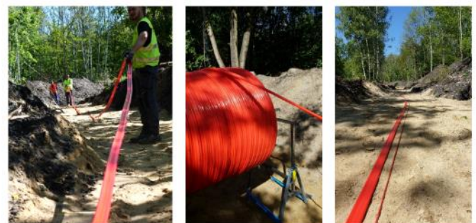
Figure 17. Distributed displacement sensors (3DSensors) during the installation within the surrounding ground.
