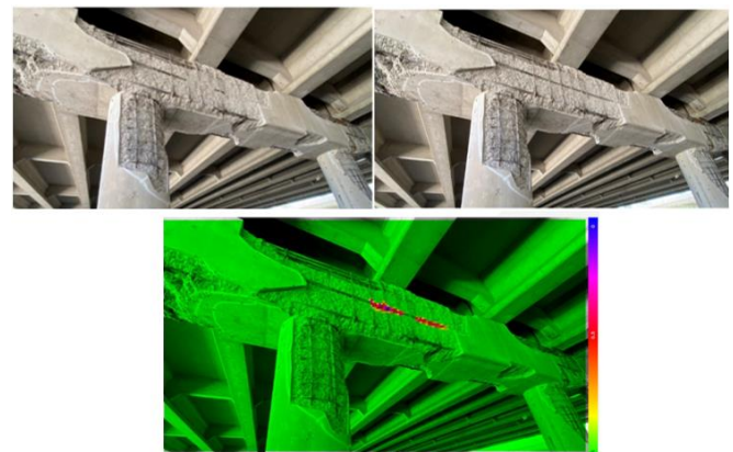
Figure 18: Example of monitoring of cracks evolution in a viaduct; the image below shows the result of change detection analysis.
