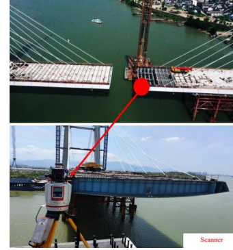
Figure 2. Tested bridge for closure in construction
