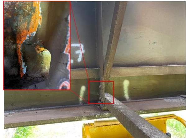
Figure 3 Monitored position with the suspected crack at the welded connection of the transverse stiffener to the main girder web plate
