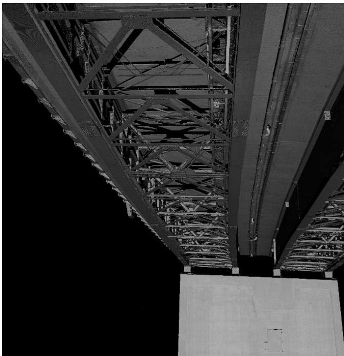
Fig. 4: Extract from the 3D point cloud of span 7 of the motorway bridge. Intensity values are shown as grey scales.
