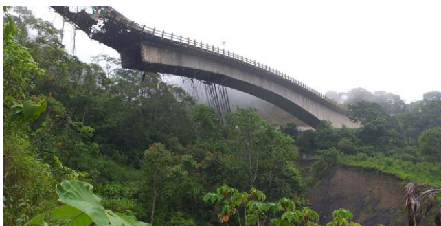
Figure 6. Los Grillos bridge structural collapse.
