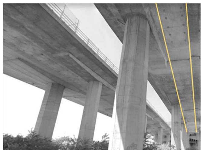
Figure 1. Two in-parallel motorway steel reinforced concrete viaduct. Yellow lines show extended deck interface.
