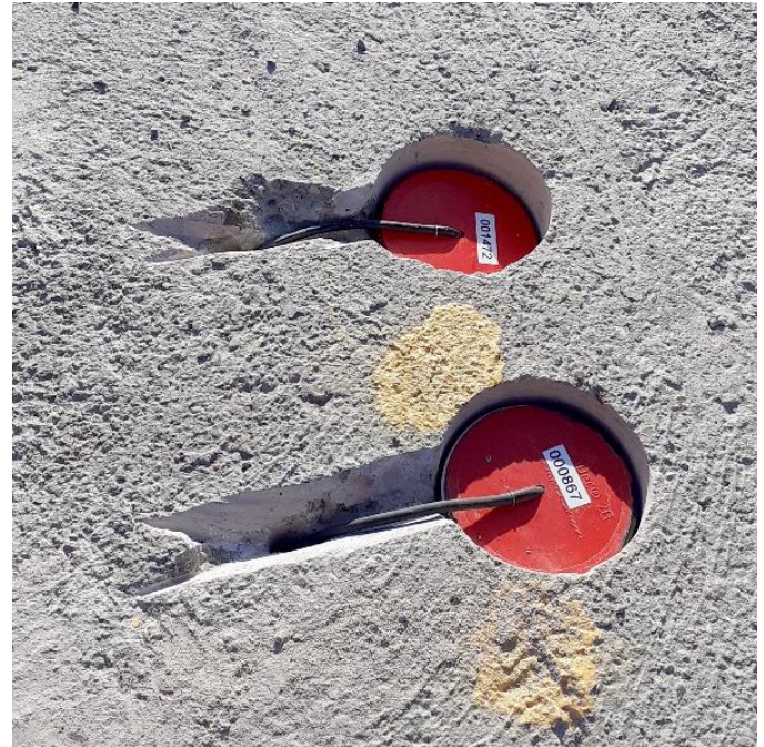
Figure 10. Installed sensors with remote antennas (Copyright: Benedikt Seuss, Infrasolute).
