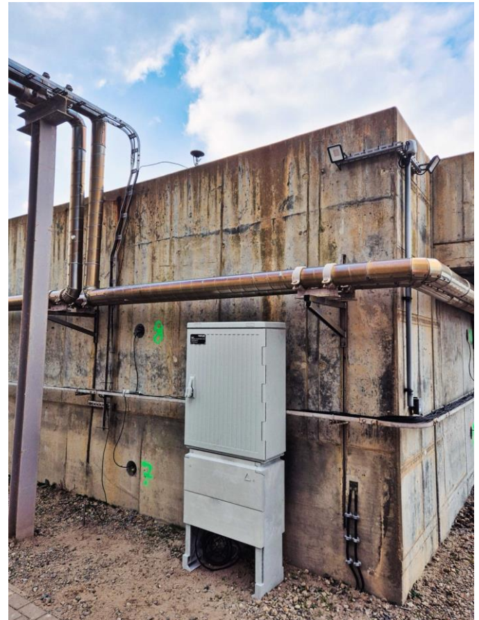
Figure 13. The monitoring computer sends all multi-sensory results (movement, leakage, corrosion) to the TEX-Sky Monitoring Cloud.
