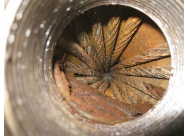
Figure 5. Corroded strands within the anchor head area.
