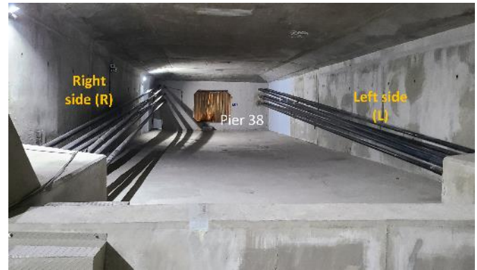
Figure 5. PSC box girder of test bridge
