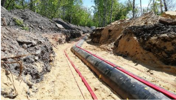
Figure 18. The view of the monitored section during final stage of installation (just before its backfilling with the soil).
