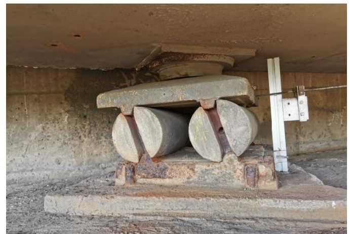
Figure 3. Monitoring system on the bridge bearing.
