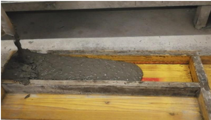
Figure 3.4 Flowing of UHPC in the 60cm length formwork (flowing time: 1min14s)
