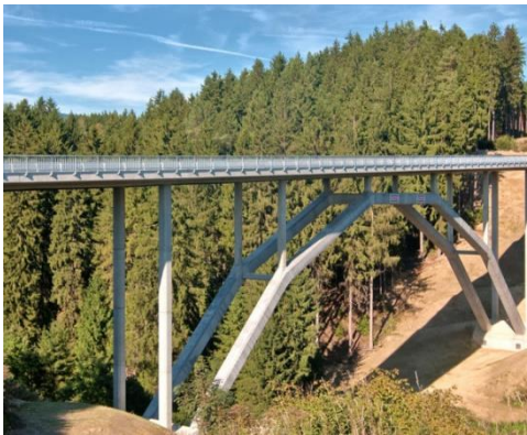
Figure 1.5 WILD Bridge in Austria [23]
