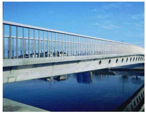
Figure 1.8 Sakata Mirai Footbridge [30]
