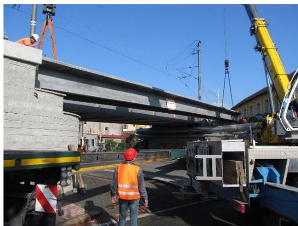
Figure 2 Installation of the UHPC beam in Tabor
