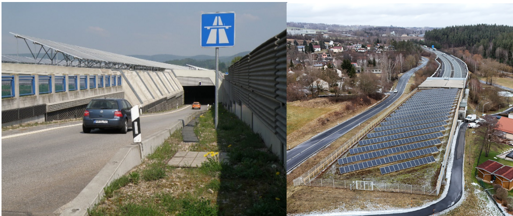
Figure 3: PV-modules on noise protection tunnels (photo: left: BASt, right: Autobahn GmbH, NL Nordbayern)
