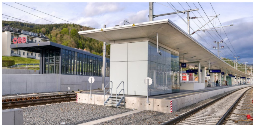
Figure 5: Station Mürzzuschlag, platform 4/5
