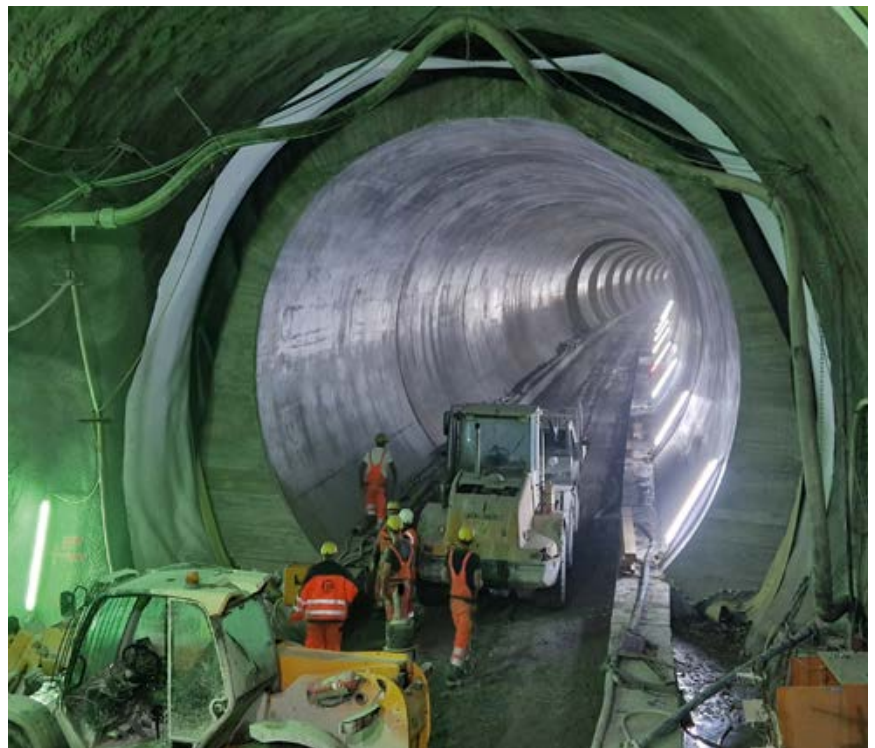
Figure 3: Concrete in tunneling, here Semmering Base Tunnel.
