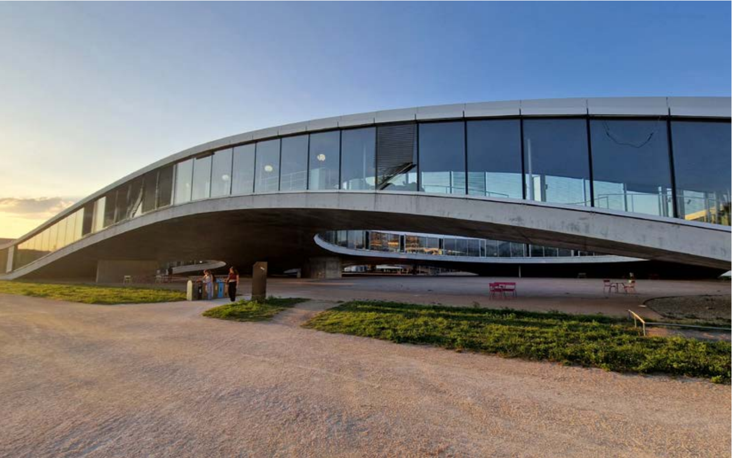
Figure 1: Extreme slender concrete structures for architectural reasons but also to achieve record-spans of bridges.
