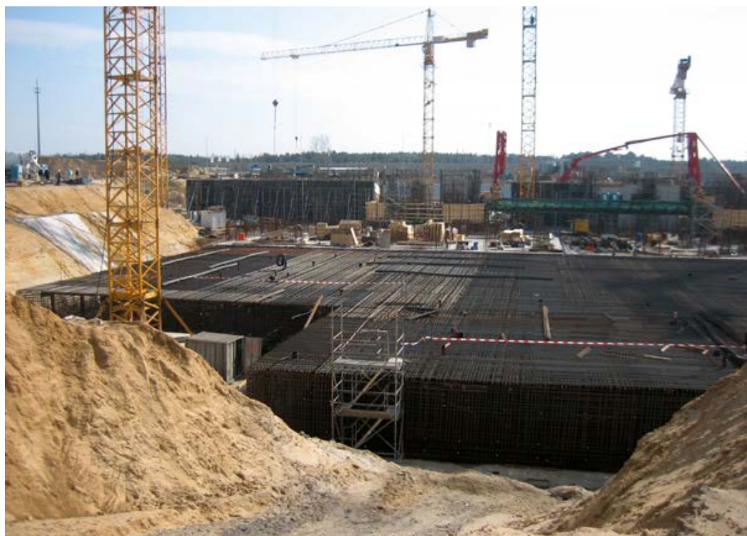
Figure 5: Reinforcement cage of 3.8 m thick ground slab.
