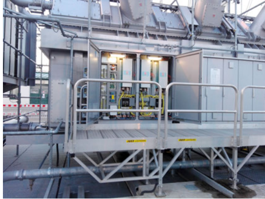
Figure 2.29: DCC cabinet at 400/110/30 kV 300 MVA transformer.
