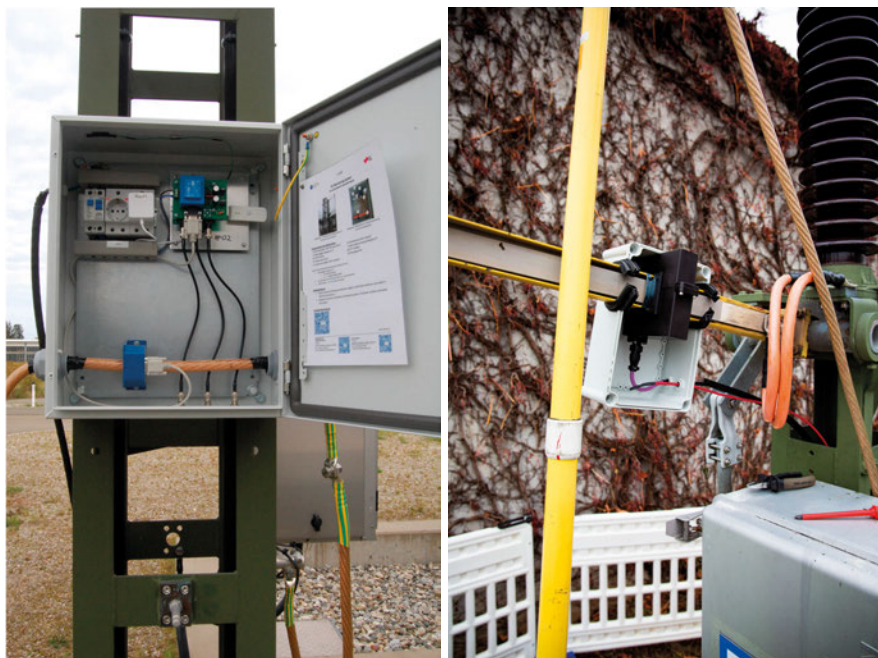
(a) Installed transformer neutral point current measurement system with open cabinet. (b) Split-core CT installed on a transformer neutral point switch with the cabinet and temperature sensor.
