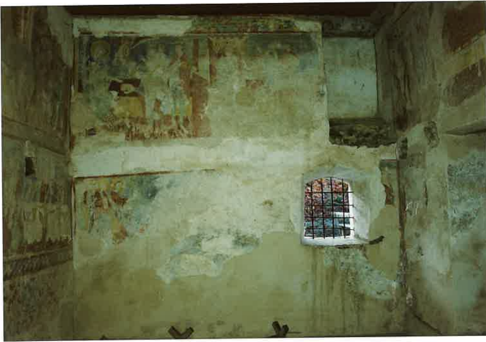
118 Hocheppan, Kapelle, Blick zur Westwand
