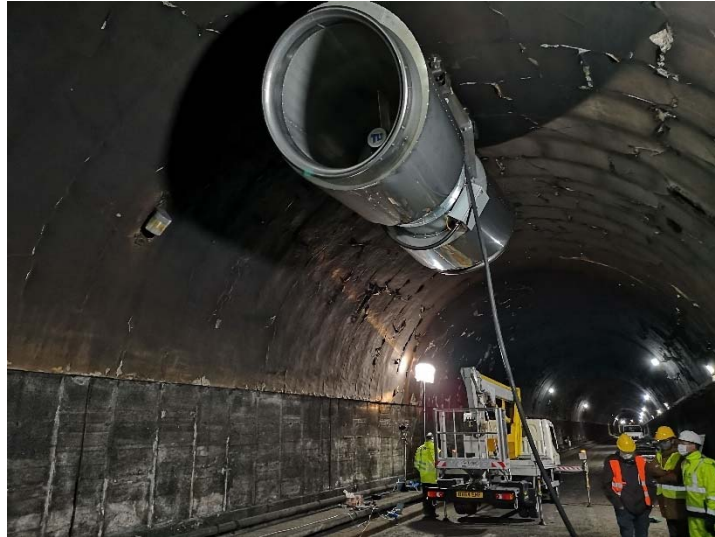
Figure 3: MoJet installation in the Rendel Street branch tunnel
