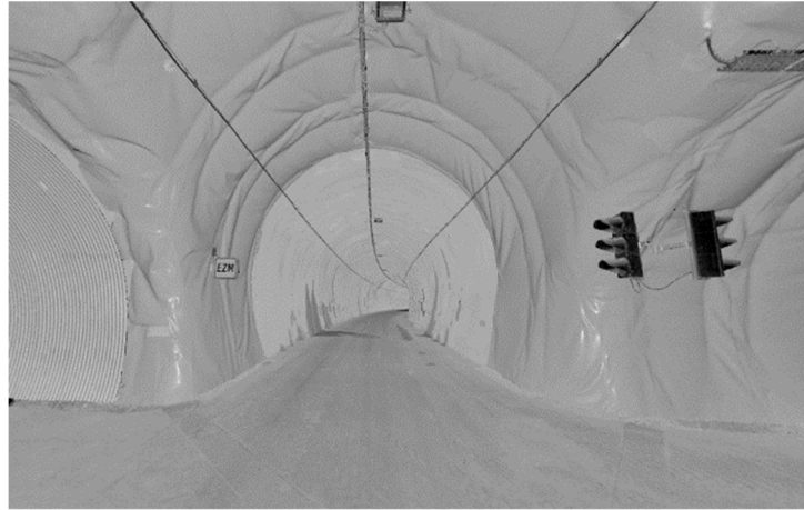
Figure 3: Laser scan data by RIEGL at ZaB
