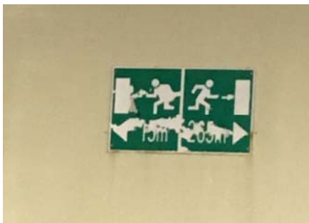
Fig. 3: Example of a faulty escape route indication sign
