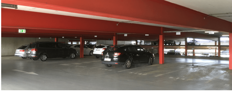
Figure 2: A photo showing the parking deck where the measurements were conducted. The position from where this photo was shot is indicated in Fig. 1 with a camera icon.
