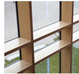
[Abb.141] Pfosten-Riegel-Fassade
