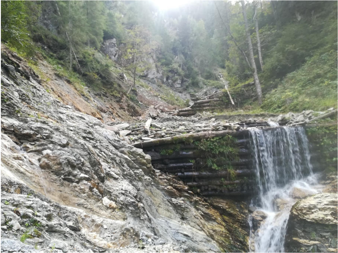
Figure 6-39: Check dams in torrent segment 7 at appr. 980 m: Check dams act as sediment-restraining barriers and limit the capability of the torrent to mobilize compartments of the torrent bed.
