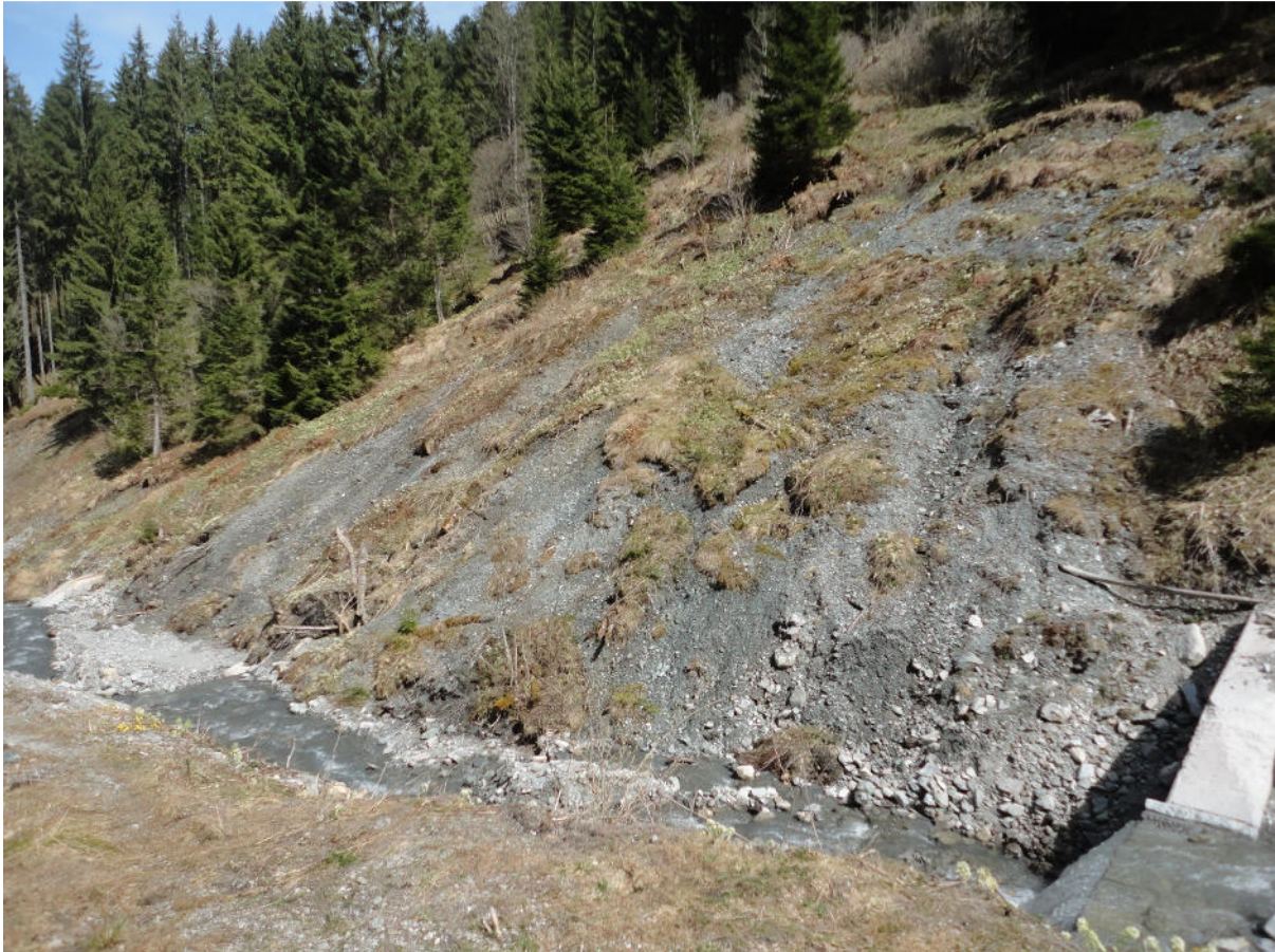
Figure 6-40: Landslide body at the E side of torrent segment 7 (Lorenzerbach) at appr. 920 m. Compared to the area that is affected by the landslide, its contribution of material is rather low.
