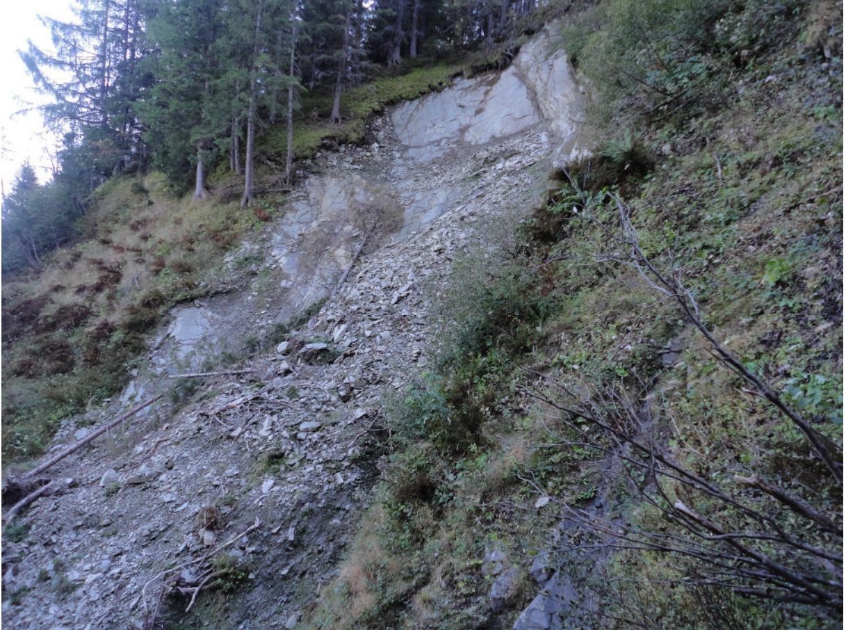
Figure 6-18: Discontinuity-controlled failure mechanism exposed on the southern slope of the Lorenzerbach at appr. 1450 m above sea level. Fragmented material accumulates towards underlying torrent. Trees can also be found in the landslide deposits.
