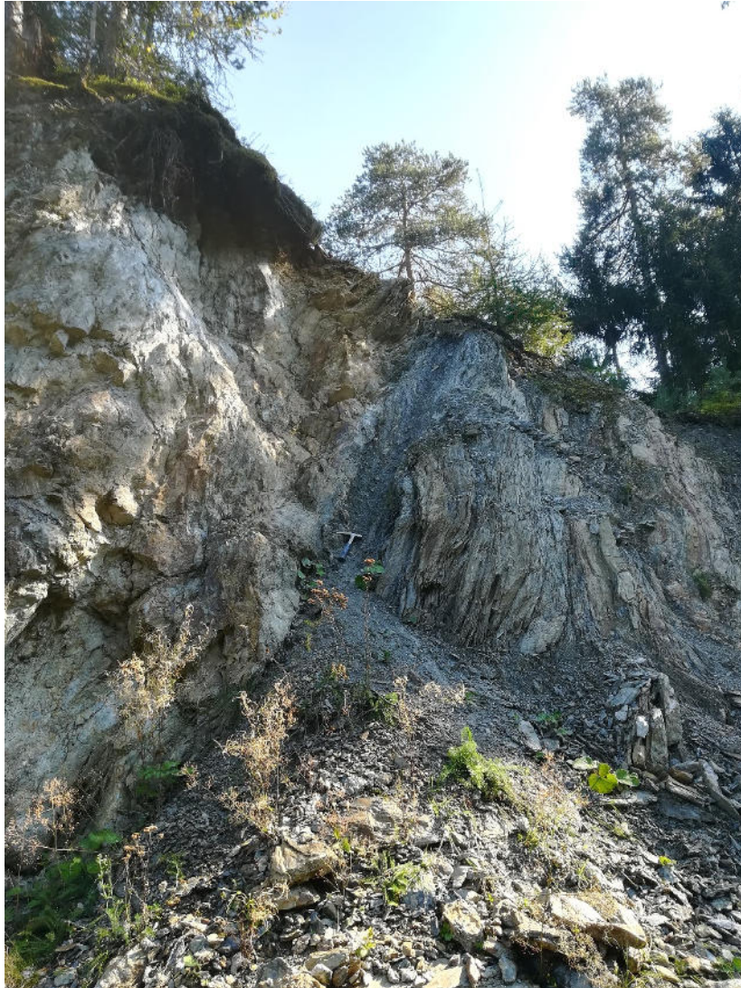
Figure 6-1: Folded greywacke schist with an ~80 cm thick, northwards dipping fault at an outcrop along a forest road to the E of the Lorenzerbach in the lower study area.
