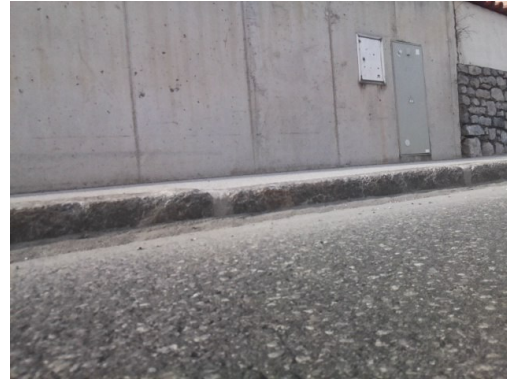
Figure 5.24: Wall behind pavement edge
