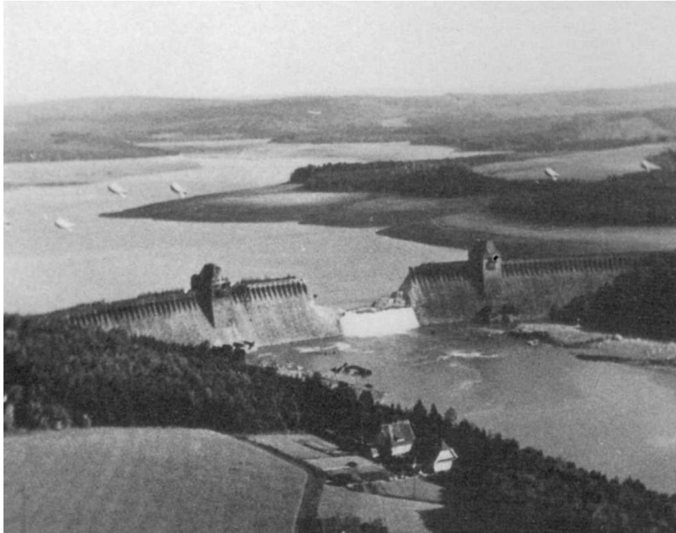
Figure 2. 3: Möhne dam failure (Wikipedia)
