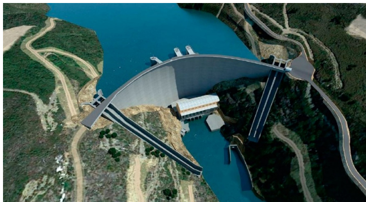
Figure 1. 1: Hydropower arch dam (iagua, 2017)
