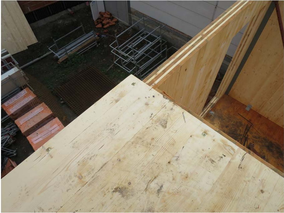
Figure 5.18: Mounting of the ceilings using screws
