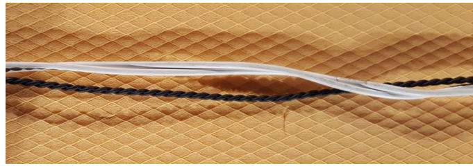
Figure 3.8.: Comparison of the tightly twisted pair cable (black, r_w = 0.42 mm, s = 1.5 mm) and the non-twisted audio cable (white, r_w = 0.62 mm, s = 2.8 mm) used for the measurements of Table 3.3
