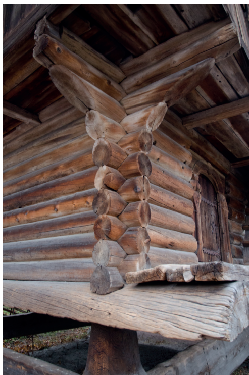
Ill.88 Corner detail, Tveito loft
