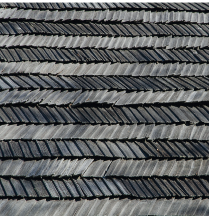
III.29 Alternating shingle roof
