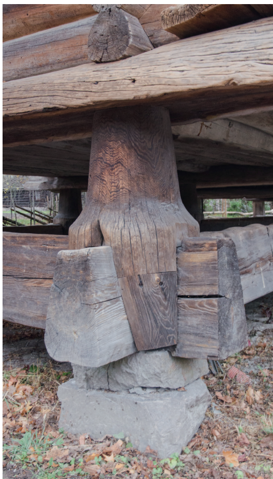
Ill.89 Foundation detail, Tveito loft
