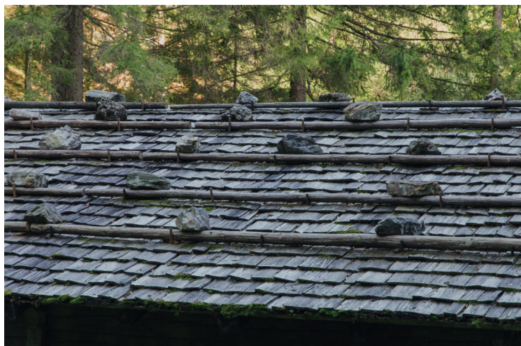
III.27 Laid shingle roof, Stübing
