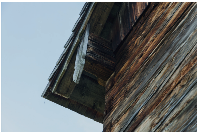
ILL.96 Protruding purlin, Kellbauernkasten
