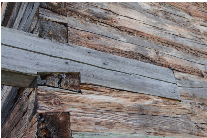
ILL.95 Balcony structure integration, Kellbauernkasten
