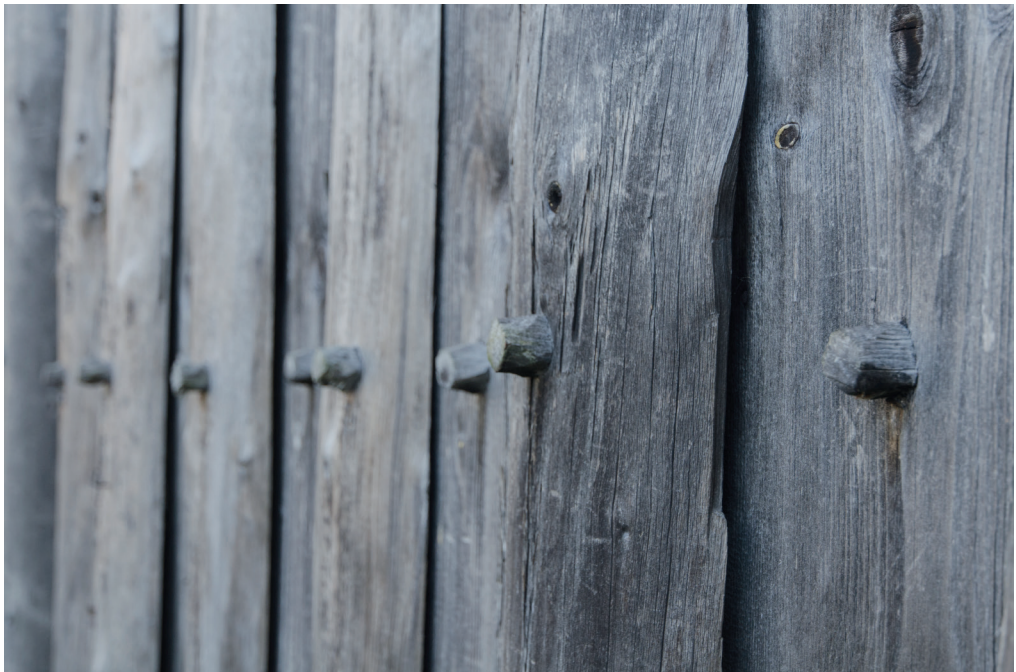
III.34 Board cladding and wooden nails, Salzburger Freilichtmuseum
