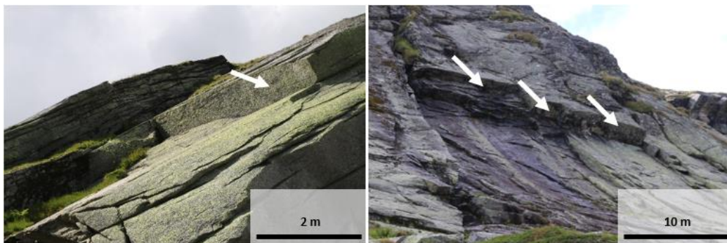
Figure 49 Photographs of Joint Set 3 characteristics.
